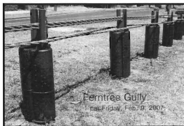
Photo 2 : Wire rope barrier after
