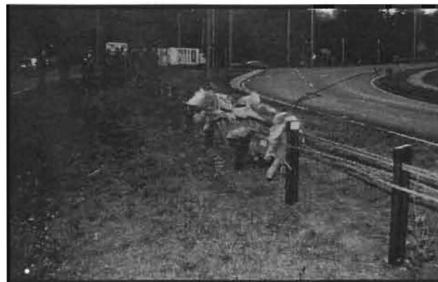
Photo 1 : Wire rope barrier before
